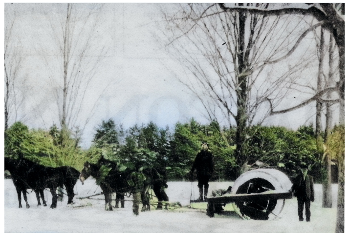
In 1923, snow rollers were used to keep the winter roads open. Arthur Sanborn is driving with Ingalls behind the roller, the gentleman besides the rear horse is not identified.
